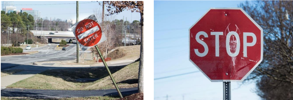
Figure 1.4 Example of damaged Signs: Non-aligned and Spray Painted
