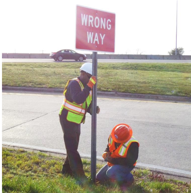
Figure 3.5 Crew Members Installing a Wong Way Sign
