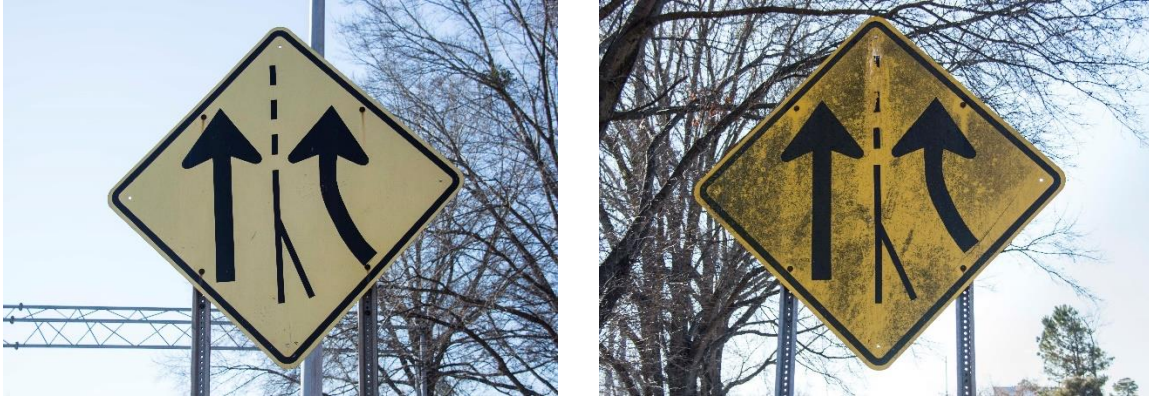
Figure 1.3 Example of Deteriorated and Damaged Signs: Faded and Tree Sap Content
