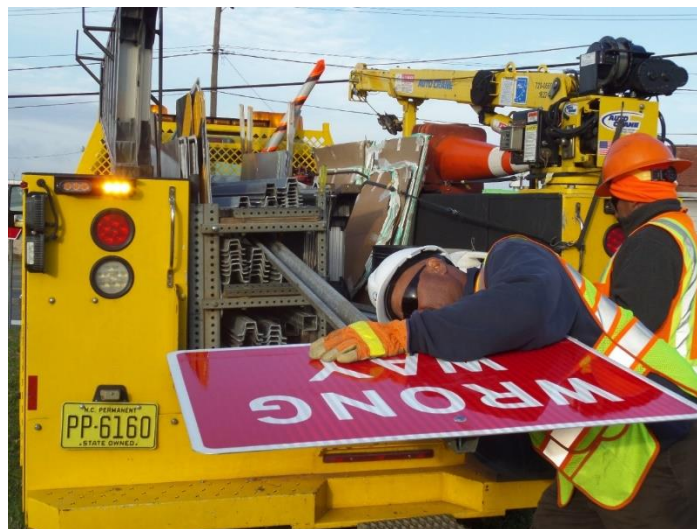
Figure 3.4 Assemble of a Wrong Way Sign to the Pole
